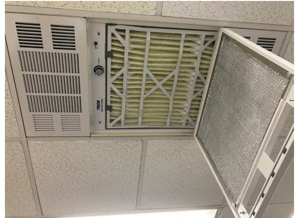
Access Door Opened
